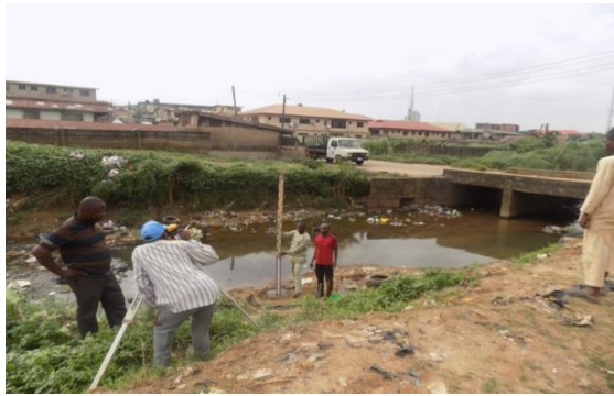
Training of Volunteers and Installation of river gauge in the river and at the river bank
