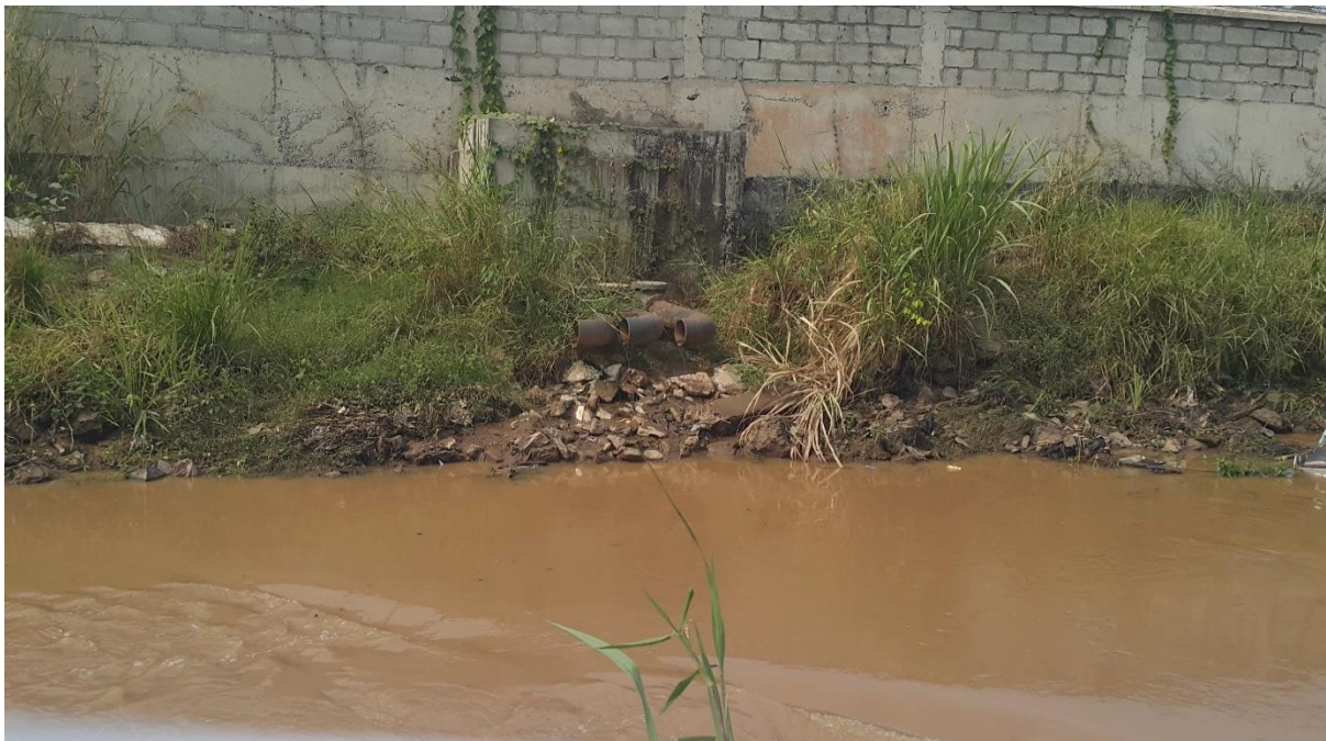
Figure 5. 11: Discharge point for industrial effluent from facilities into the river channel
