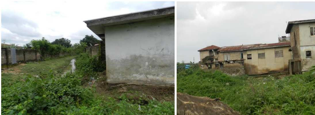
House on the setback marked in 2011 for demolition, Odo ona, orogun,
